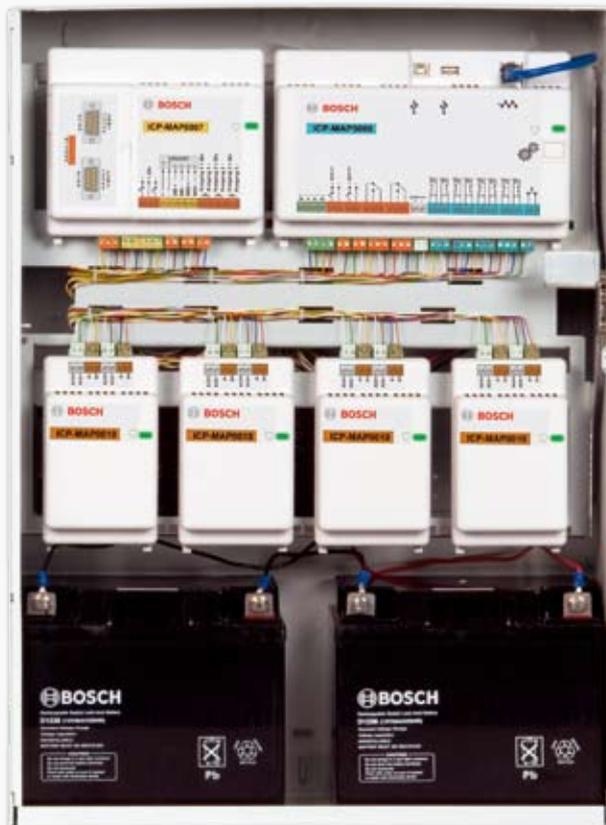
The Modular Alarm Platform 5000 system components are well arranged and mounted inside the robust metal housing to provide maximum safety to the installer and the user.
